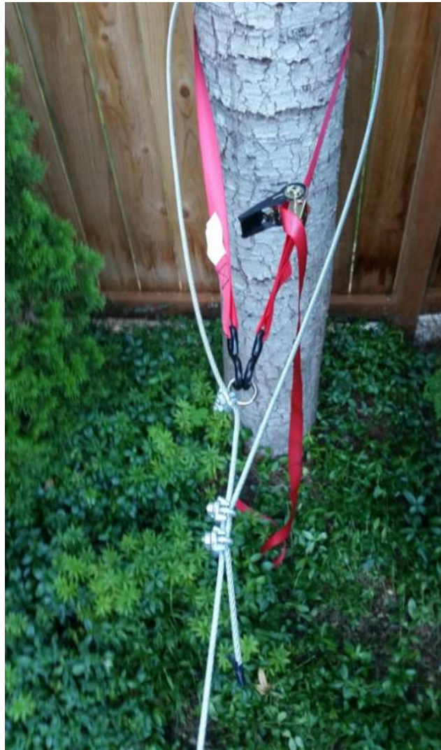
Ratchet Strap and Welded Ring Cable Tensioning Method
